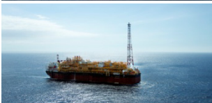
CLOV FPSO / TOTAL
